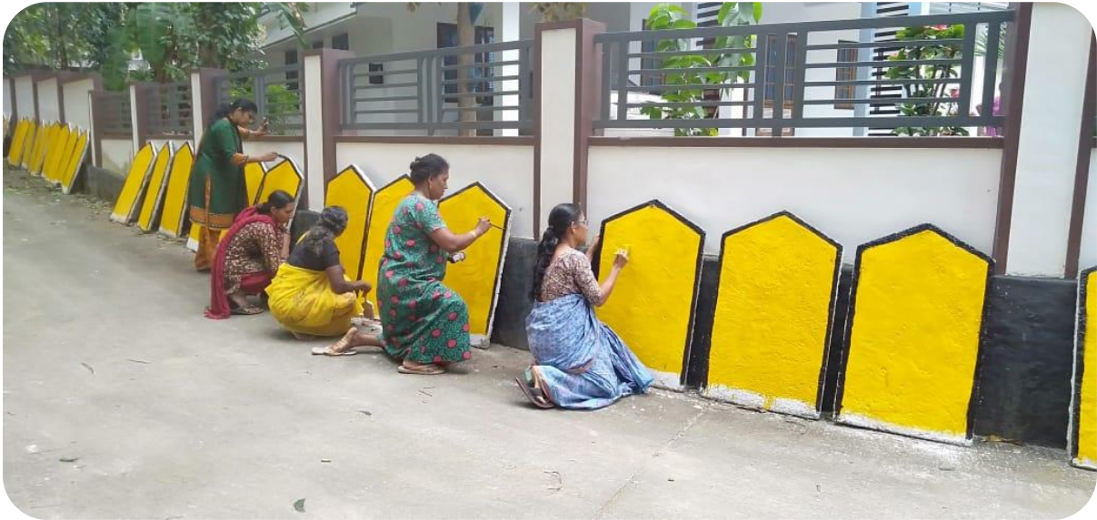
Construction Group Engaged in MGNREGS Board Painting Work
