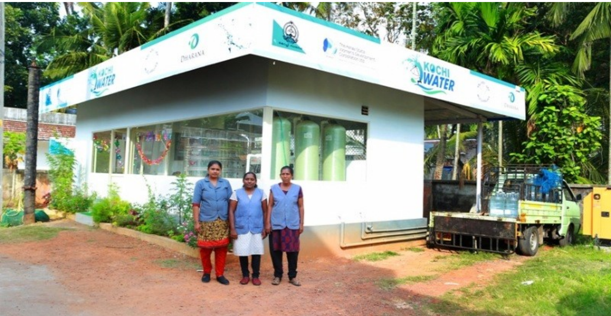
Reverse Osmosis plants
