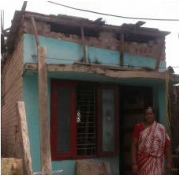
Can see the old painted wall in the photo.
